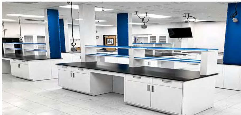
UTILITY CHASE - REAGENT SHELVING - RACEWAYS
